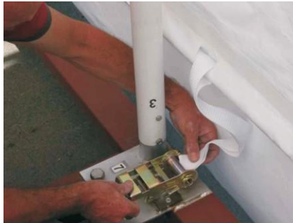
Installing ratchet straps
